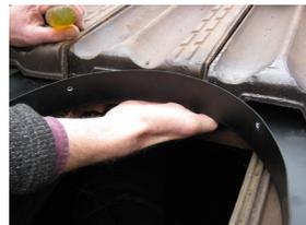
6. Lift flashing up underneath the tile using the hand to ensure wind driven rain cannot make its way up under the tile above the flashing.
