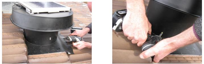
15. If a thermostat is fitted—connect the thermostat. The adjustable thermostat is connected by separating the black and the red fan wires and inserting the thermostat in the loop. The red fan wire is connected to the red wire from the thermostat and the brown solar panel wire is connected to the black wire from the thermostat. Should the wiring become undone on your adjustable thermostat the blue wire goes to terminal 1 and the brown wire to terminal 3.
