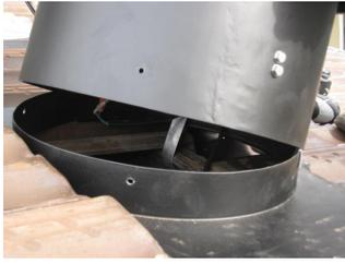
2. Locate a suitable position for the Solar Whiz. i.e. Free of shading and normally high and central on the roof for optimal performance
