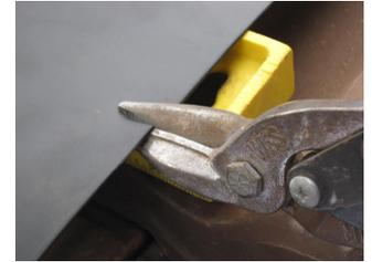
8. Shape sides of flashing to fit profile of tile. Gently tap sides for a tight fit. **Trick:** Cut flashing as shown in photos, when pushing down over tile profile.
