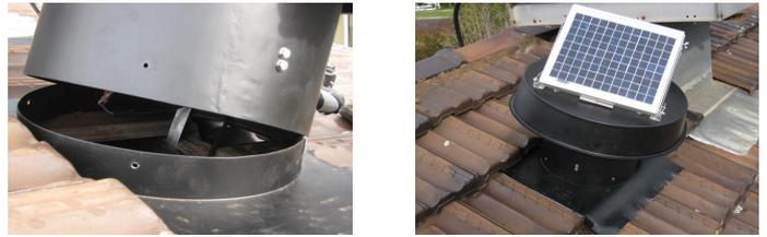
14. Use the predrilled holes in the fan housing for guiding the self cutting screws to fix the fan housing to the flashing. For extra strength, also put a screw through where the aluminium straps sits between the fan housing and the flashing.
