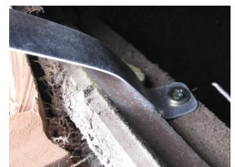
10. After the flashing has been securely fastened, silicone inside contact point between flashing and upper part of tile and the outside edge.
