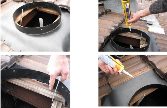
11. Silicone contact point where flashing touches higher point of tile. Do not silicone drainage valley on tile.
