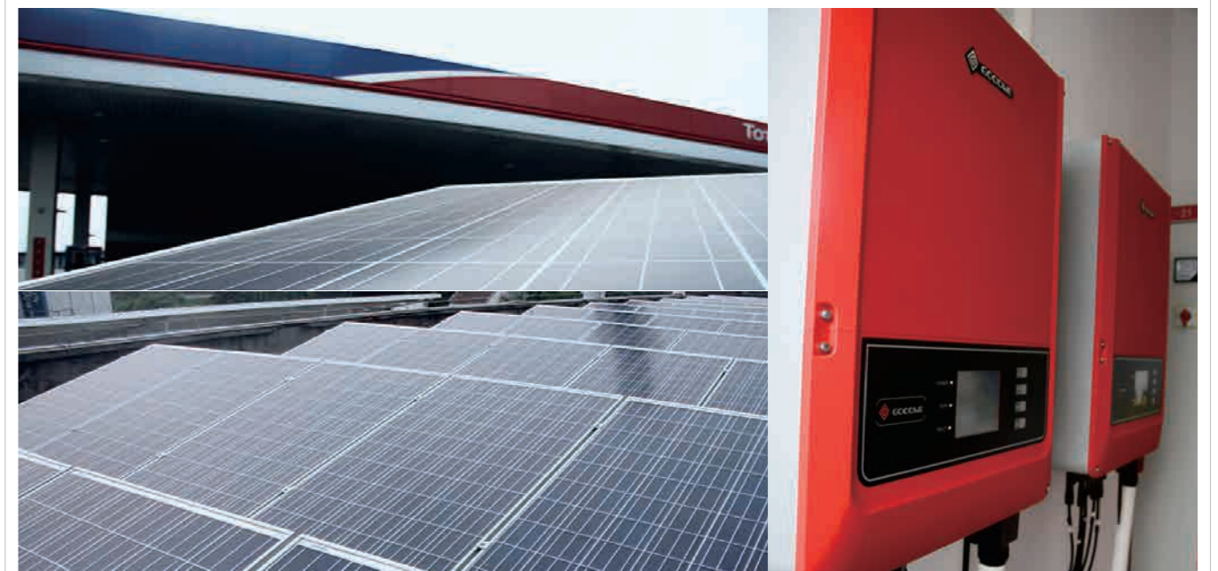
30kW, Petrol station
