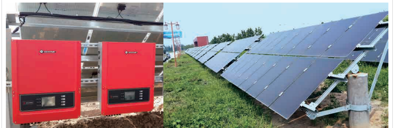
250kW, Shangdong, China
