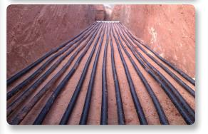
Manifold in 125mm PEH pipe at either end for connecting the inlets and outlets to the polypipes.
