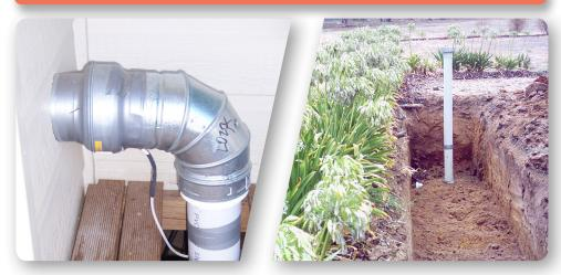
A total of 200 meters of corrugated 25mm plastic pipes (24 8m parallel lengths plus extra) ensures the heat exchange between the air and the around.
